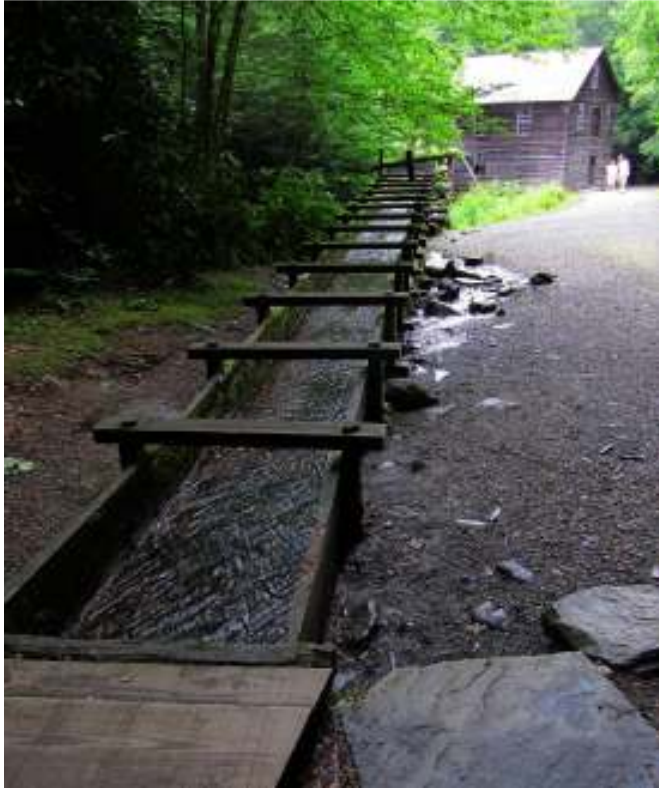
Typical Mountain Community Mill with Raceway
